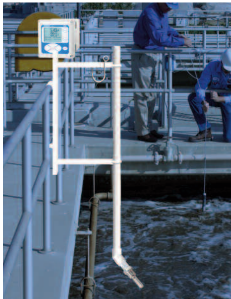
Figure 26. Photo on left shows sensor being dangled into the pond, an incorrect installation. Photo on right shows correct sensor mounting – sensor is threaded into a pipe conduit while cable is run through the pipe of the Handrail Mounting Assembly.
