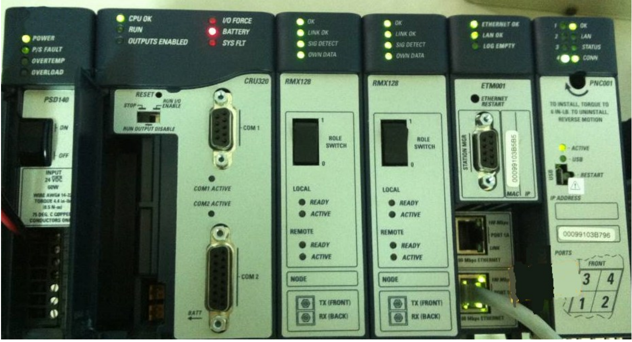
Figure 154: Rack Configuration for this Application
